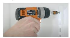
Fasten the wallband with a screw in the upper hole.
