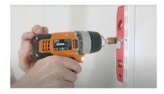
Preferably, use a leveller in order to determine that the wallband is straight, before fastening the other screws through the holes in the wallband.
