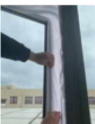
5. Attach the narrow side B (zipper closed) from the center to the left and right or up and down on the casement.
