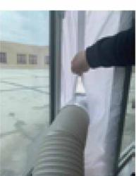
6. Open the window slightly and pull out the vent hose through the Window sealing kit using the zipper.
