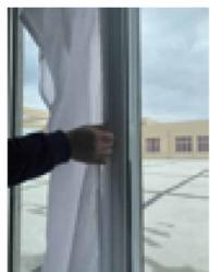
3. First attach the wide part (side A) of the sealing cloth (zipper closed) with the window open. Start in the middle and then attach left and right or up and down on the window frame.
