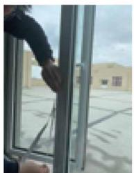
2. Attach the velcro strap to the (side A) window casement inside or outside. The side where the handle is.
