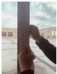
1. First open the window and clean all surfaces where the Velcro strap should be attached. Clean the surfaces of the frame and casement so there is no dust and grease. Open the Velcro tape's self-adhesive part, attach it to the window casement.
