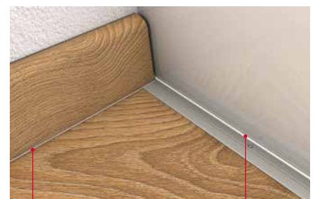
Silicone joint Silicone joint
